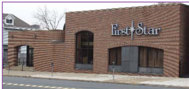
First Star Savings Bank, main branch, at 418 W Broad St. Bethlehem
